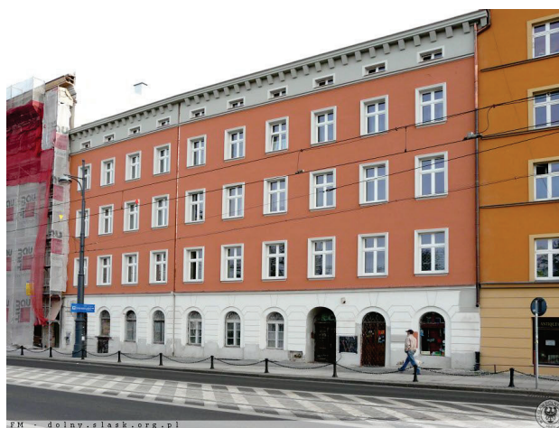
Fig. 5.1. A tenement with flats in Wrocław at Grodzka 5–6 street after renovation within the LRP in years 2005–2006. Archives from 2008. Source: https://polska-org.pl/742054,foto.html [access: 05.05.2022]
