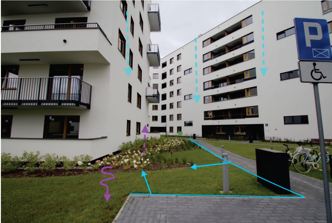
Fig. 6.12. Typical element of rainwater system at the Mickiewicz housing estate – flower bed
