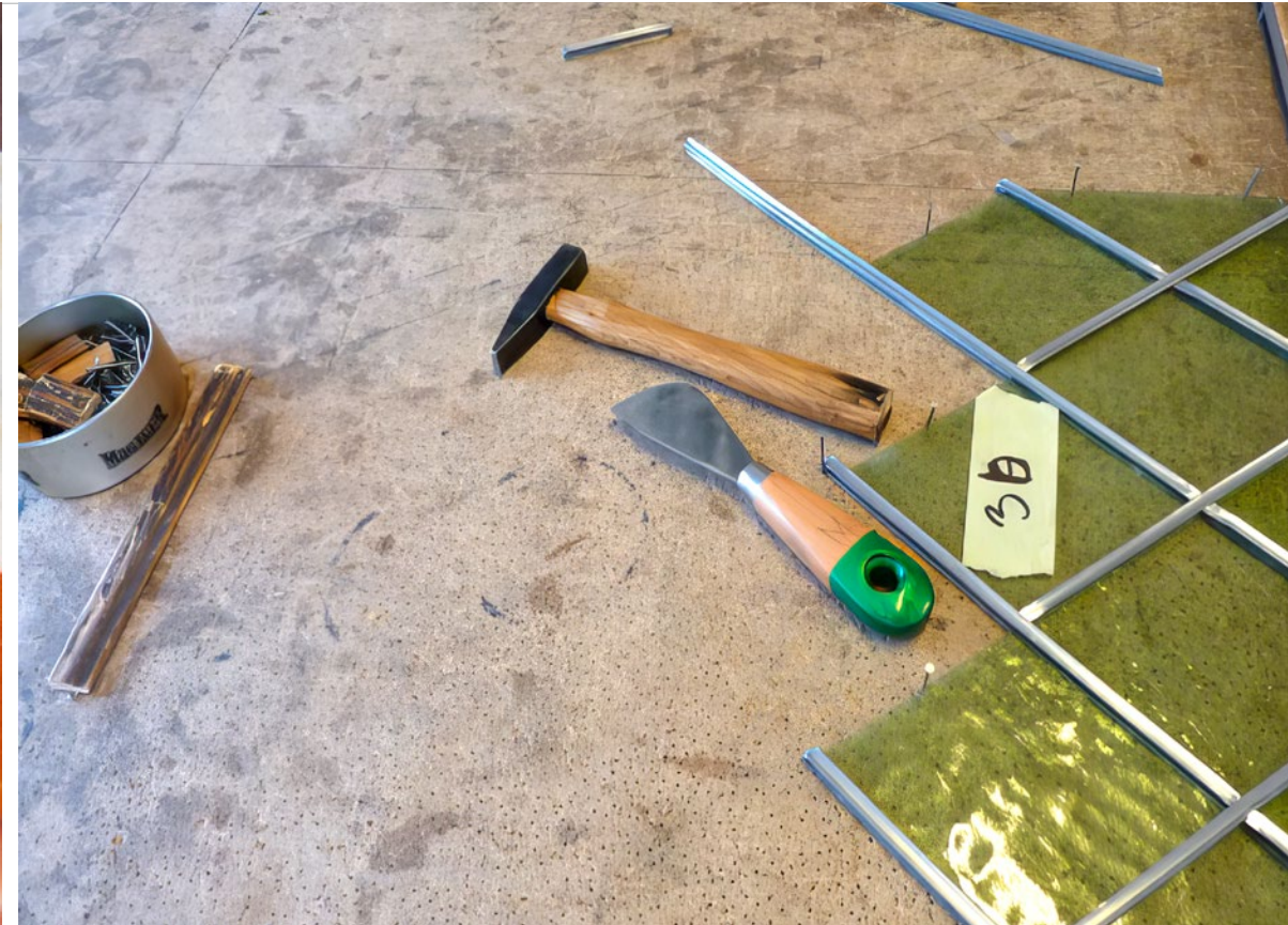
Fig. 69. Glass fitting in lead profiles
