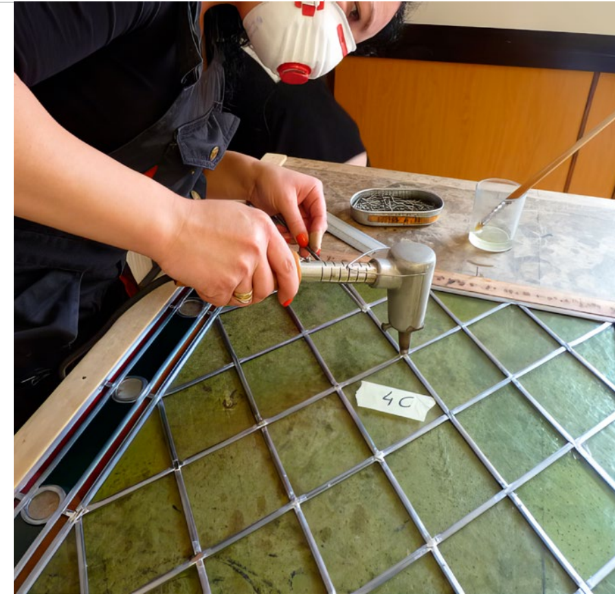
Fig. 70, 71. Soldering of lead profiles
