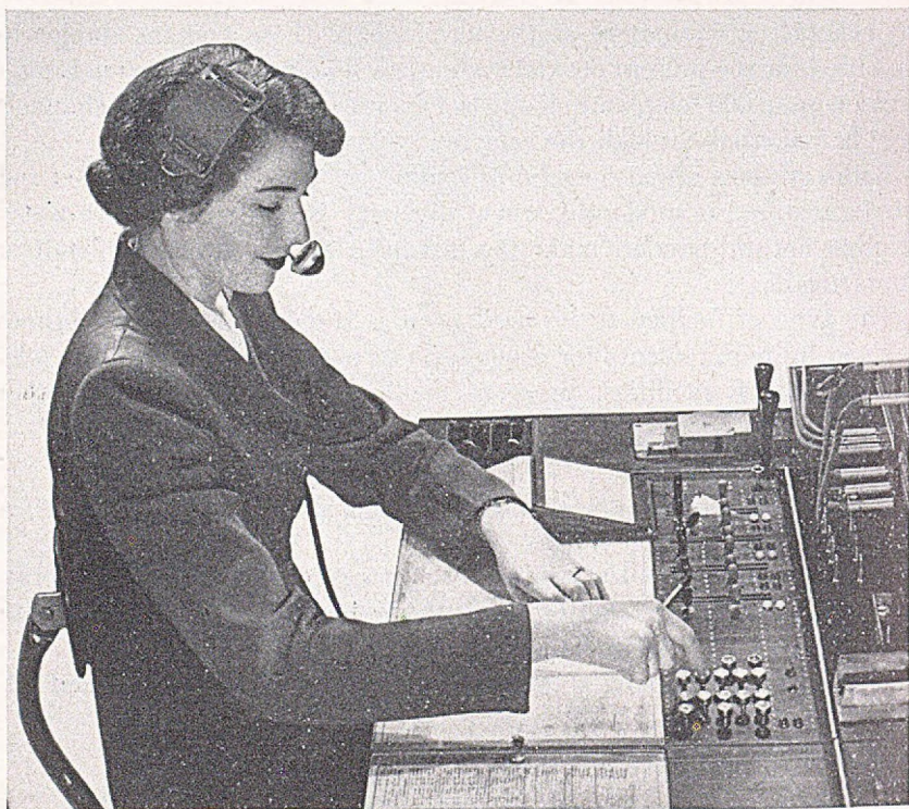
Fig. 12—Toll switchboard position with key set used for toll dialing.
