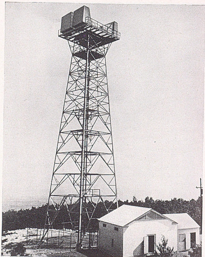
FIG. 10—Microwave radio relay tower at Cotoctin Mountain, Maryland, on a New York-Washington radio route. There are 300 message circuits in service with more planned.
