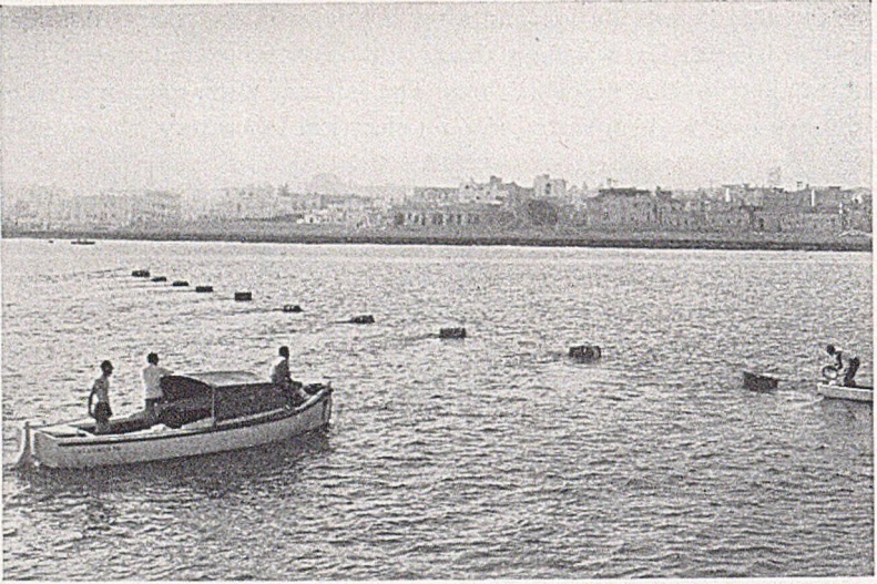
Fig. 16—Havana landing site.
