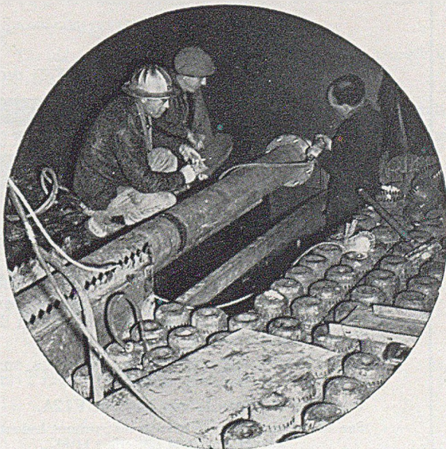
Fitting Monel tubing and bubble cap trays. (By courtesy of Messrs. Foster Wheeler Ltd.)
