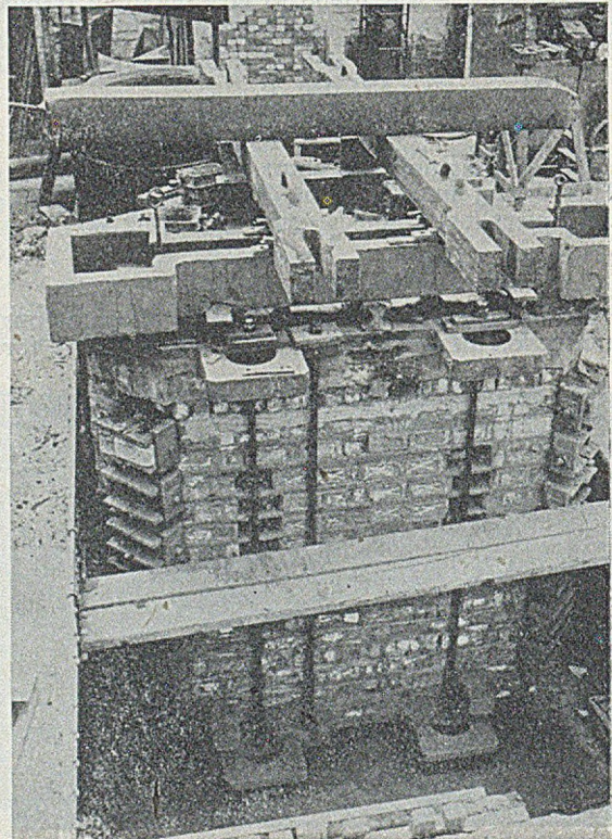
FIG. 25.—Mould ready for Casting.
