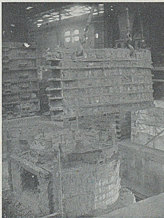
FIG. 27.—One of the Mid-sections stripped from the Casting.
