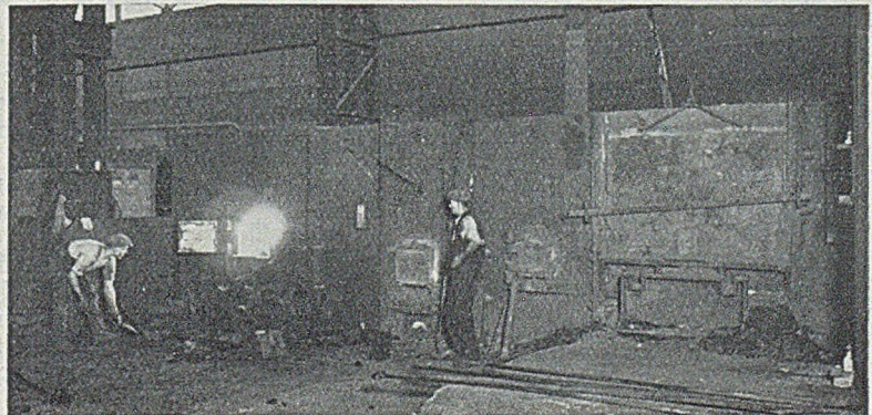
FIG. 22.—Hand-fired Reverberatory Furnace.
