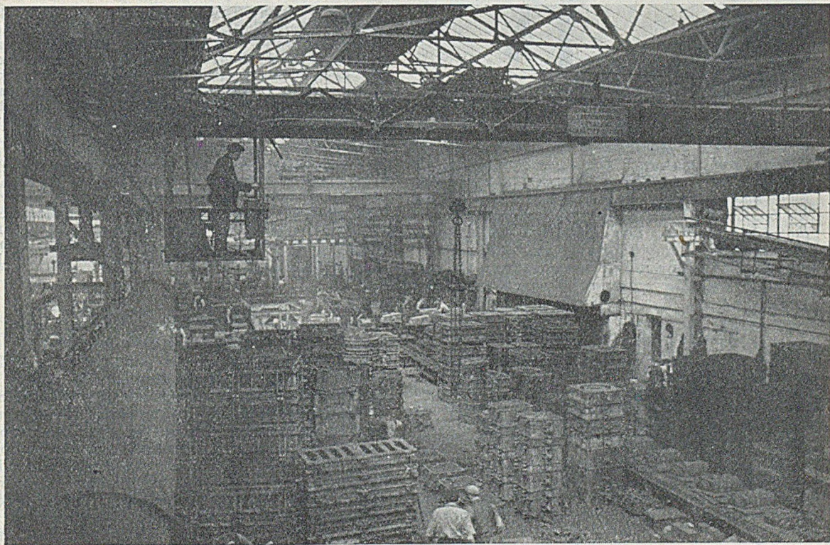
FIG. 3.—Section of the Foundry Devoted to Heavy Core making. Fume-extraction Ducts over the Entrances to the Core-drying Stoves can be seen on the Right-hand Side.
