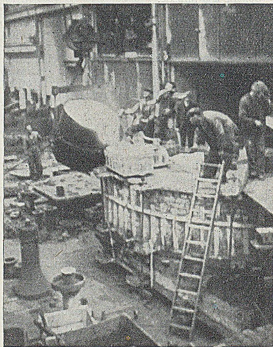
FIG. 8.—Casting the Volute Section. The Runner Box and the Method of Bolting Down the Mould can be seen.
