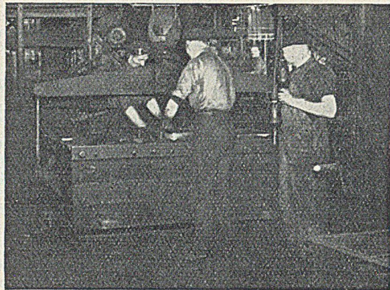
FIG. 4.—Finished Bath Mould-part (Cope) being withdrawn from a Pattern.
