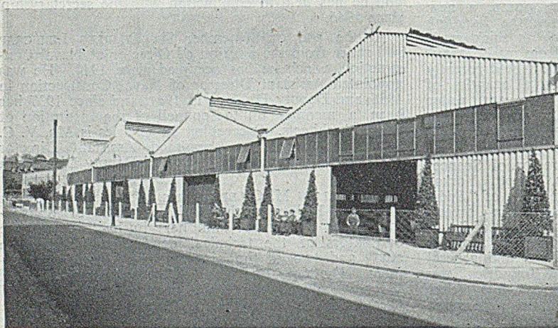
Our illustration shows the exterior of the latest extension to the foundry of the Dover Engineering Works, Limited. The decorative treatment it has received is both noteworthy and pleasing.
