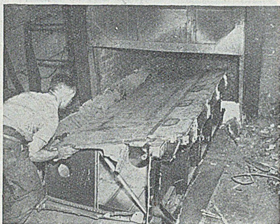
FIG. 9.—Charging a Piece of Aircraft Fusilage into a Stack Furnace.
