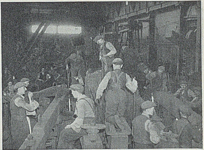
FIG. 7.—Arrangement of Binding Bars on the Top of the Mould for the Gear-wheel Casting; Rod Feeding is in Progress.
