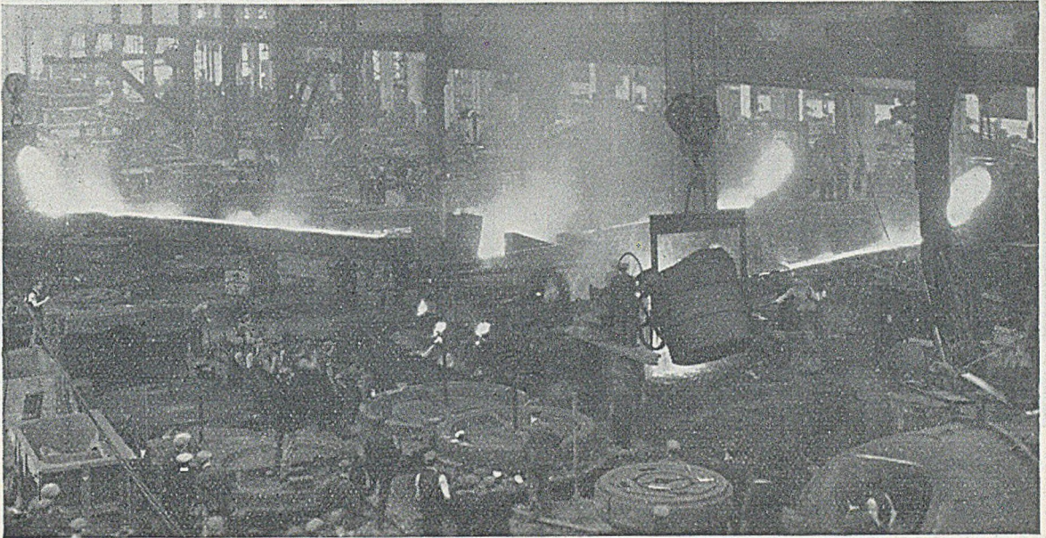
FIG. 10.—Pouring of a 75,000 kw. Exhaust Casing Cylinder weighing 58 tons; Five Ladles were employed.
