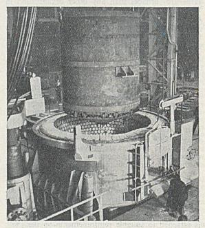
FIG. 2.—Charging Bucket lowered over the Furnace Body after Removal of the Roof. The New Furnace is lined with Metal-cased Magnesite Bricks.
