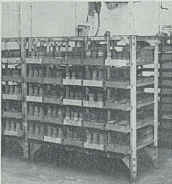
FIG. 13.—Arrangement of Stillages for holding a Large Number of Core Trays.
