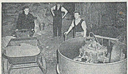
Sand from stock-pile to mixer
