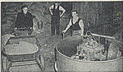
Sand from stock-pile to mixer
