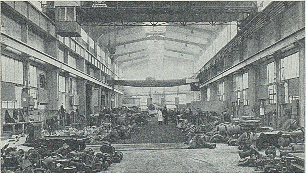
FIG. 1.—No. 2 Bay of the New Dressing Shops at Vickers-Armstrongs, Limited. This Bay is concerned with the Lighter Type of Castings.
