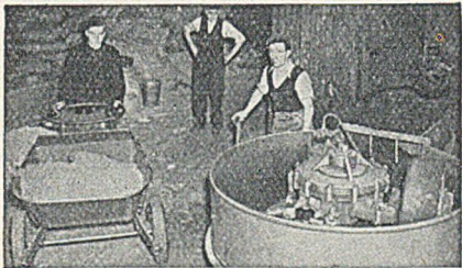
Sand from stock-pile to mixer
