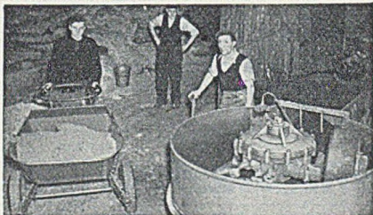
Sand from stock-pile to mixer
