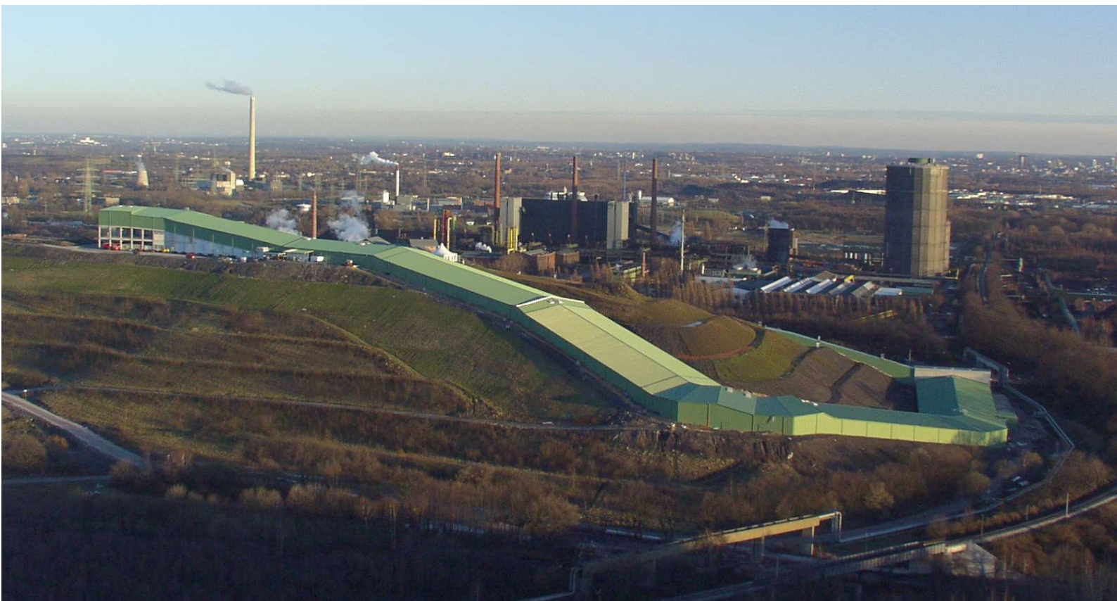
Fig. 89. Skihalle in Bottrop
