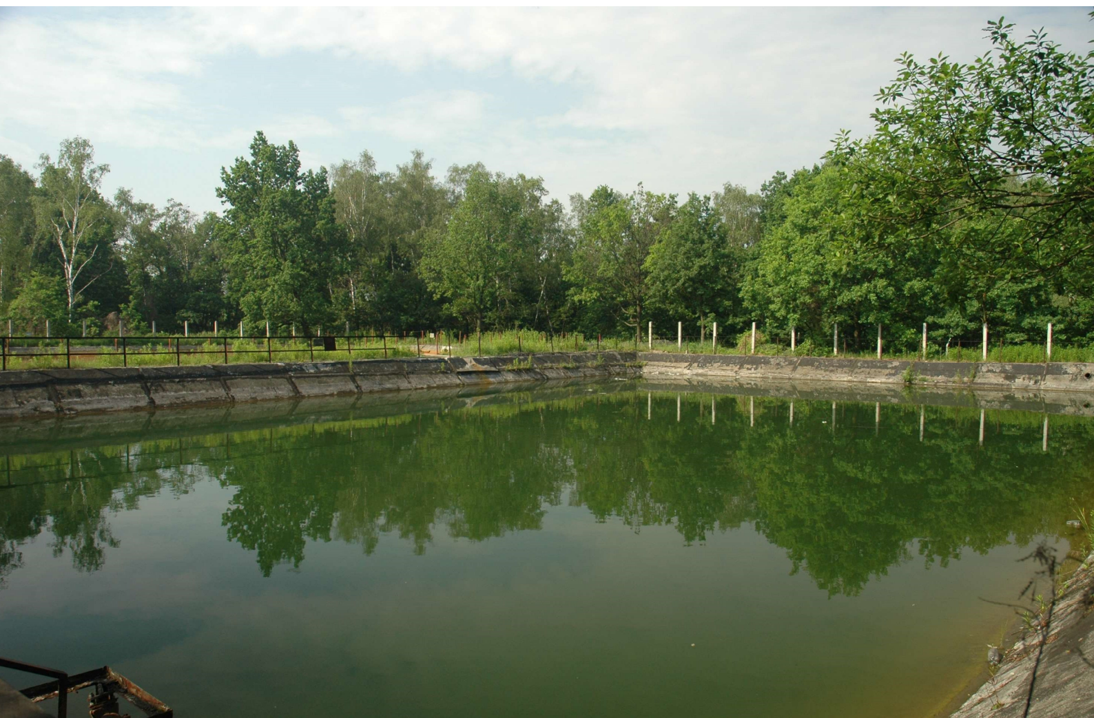
Fig. 72. Settling pond in Zabrze; photograph by A. Pancewicz
