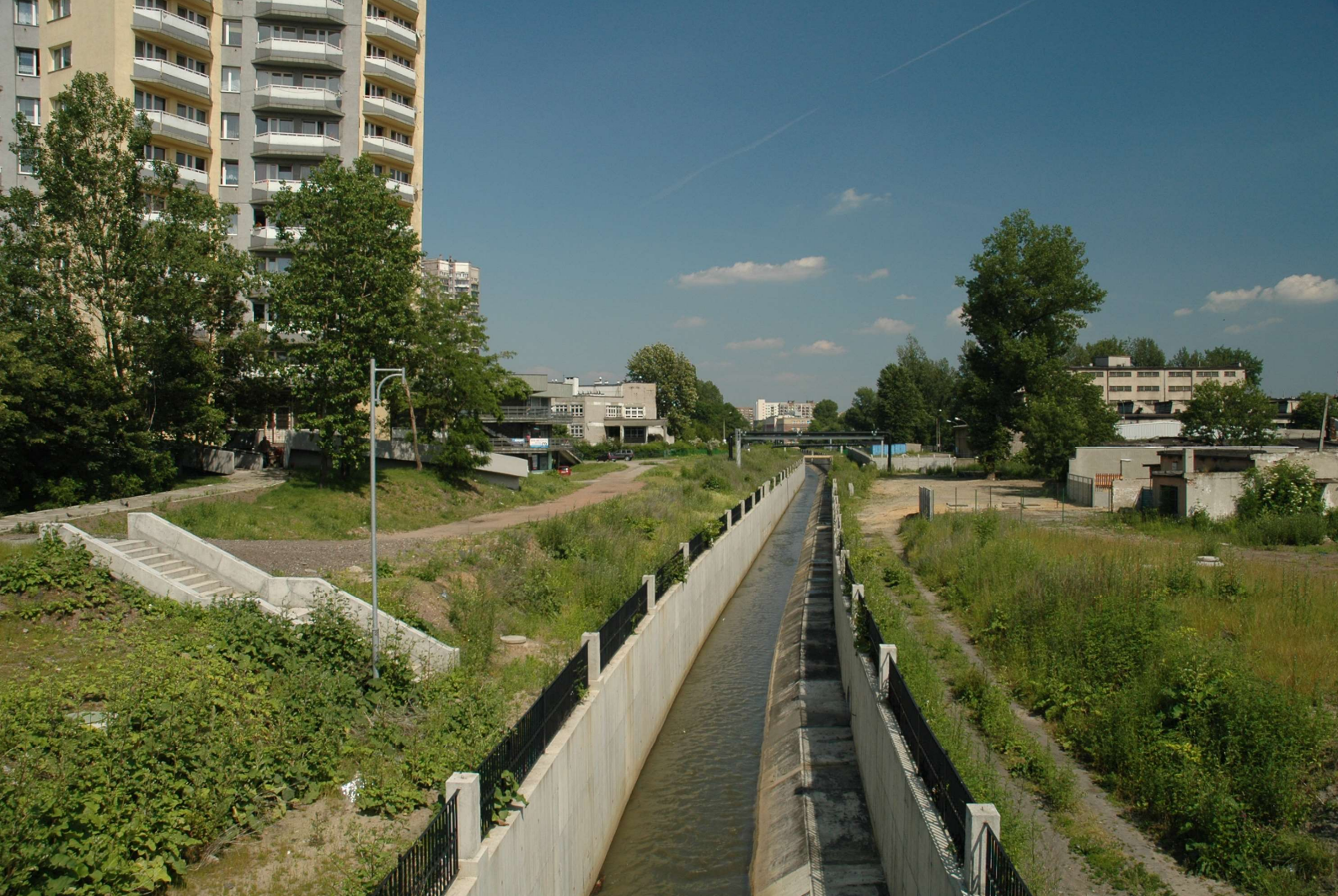
Fig. 73. The river Rawa in Katowice; photograph by A. Pancewicz
