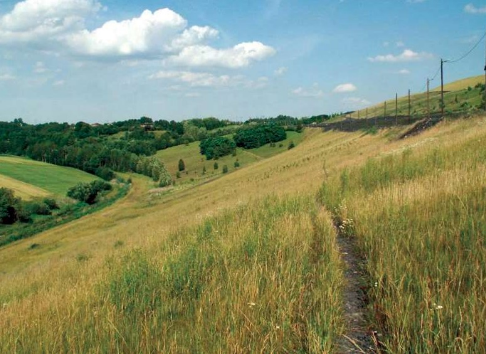
Fig. 103. First generation of measures implemented for purposes of landscape renewal. Borynia-Jar dumping grounds in Jastrzębie-Zdrój; since 1983, reclamation works have been conducted there on an area of 70 hectares, comprising such procedures as levelling of slopes and the flat top of the heap, greening by traditional methods, using fertile soil and by the soilless FRISOL method
