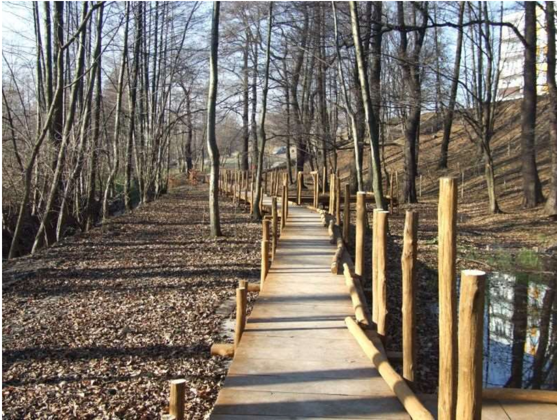
Fig. 102. Old channel of the river Słepiotka restored – a path on piles, REURIS project, 2010
