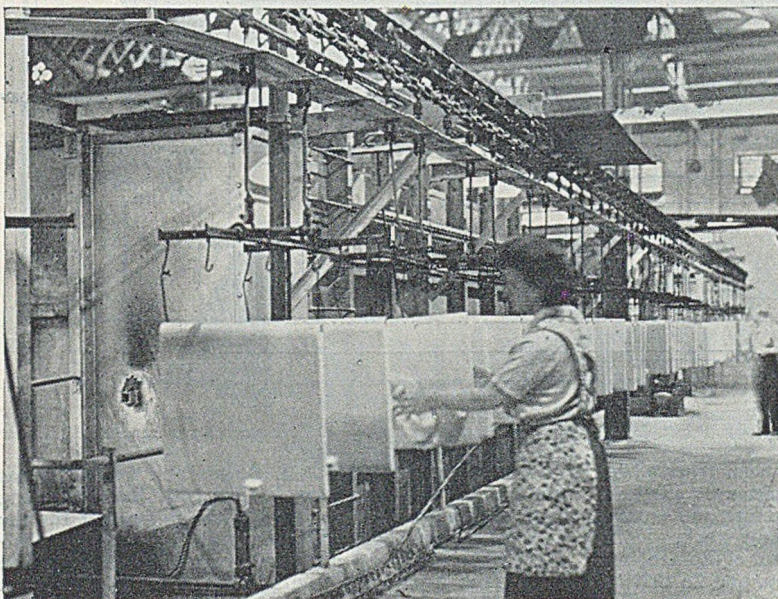
Fig. 14.—Ware being loaded on to the Continuous Furnace Conveyor.
