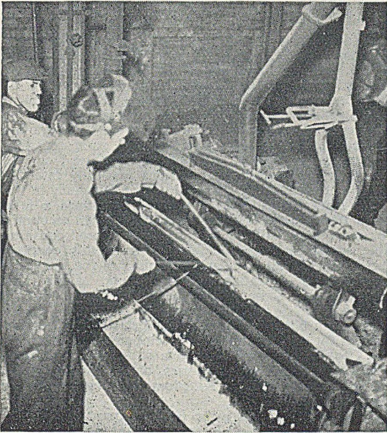
FIG. 6.—Casting, still Red Hot, being removed from the Die.
