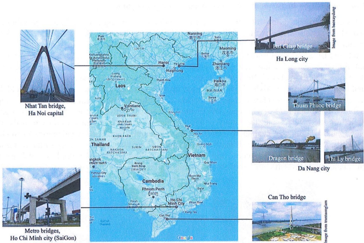
Fig. 2. SHM systems for bridges in Vietnam.
