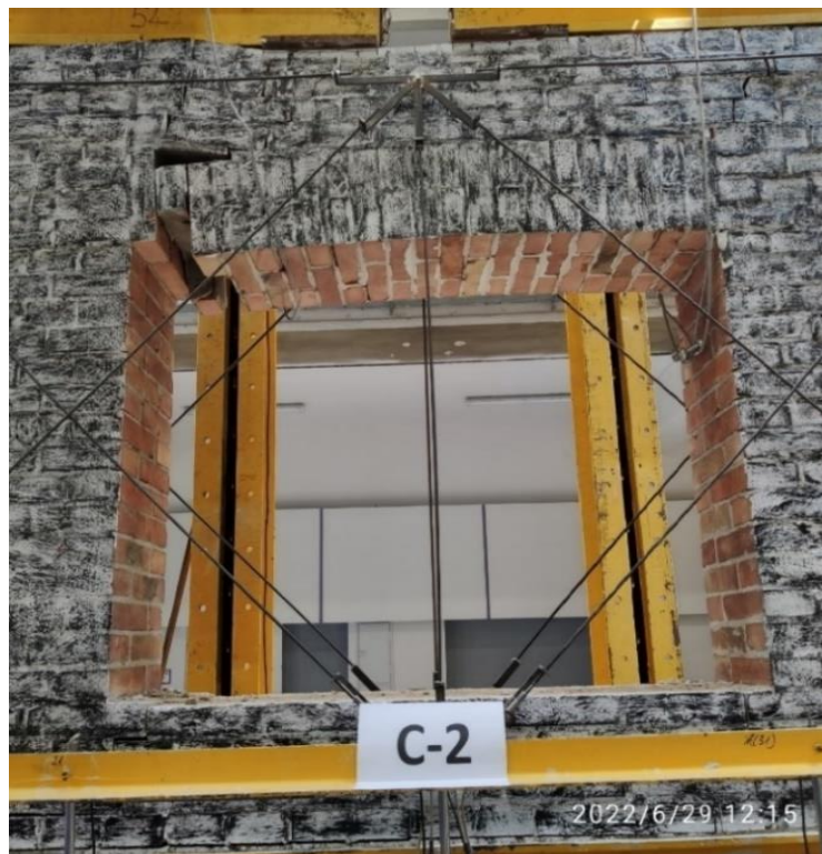
Fot. 8.4.1-4. Widok w modelu badawczego C.2 po badaniu Photo. 8.4.1-4. View in the C.2 research model after the test
