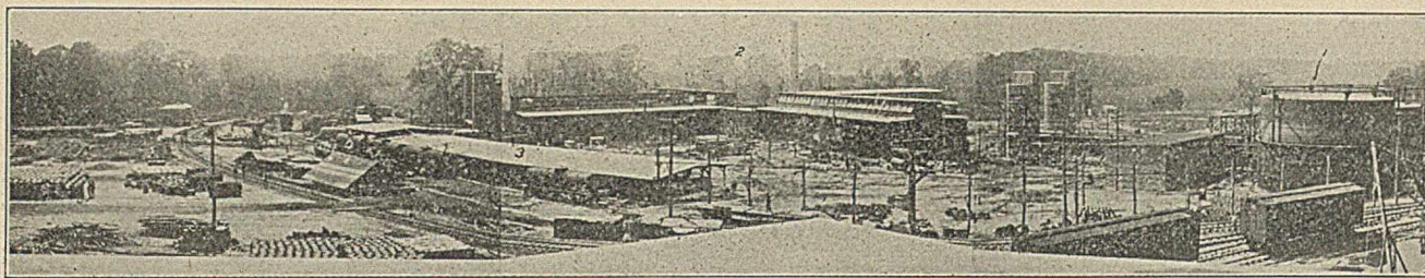
FIG. 8—GENERAL VIEW OF MUSTARD GAS PLANT
