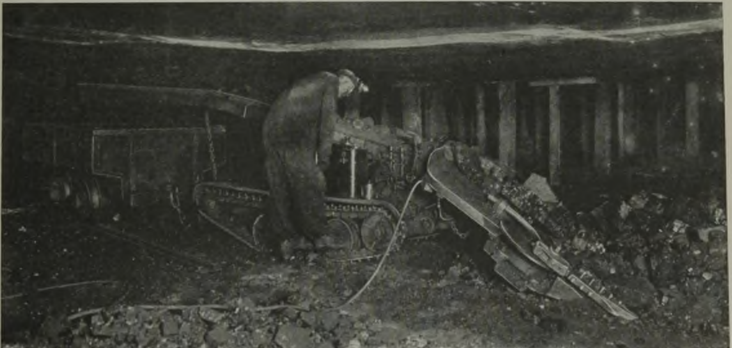
This Machine Proves Economical Though It Averages But 75 Tons a Day
