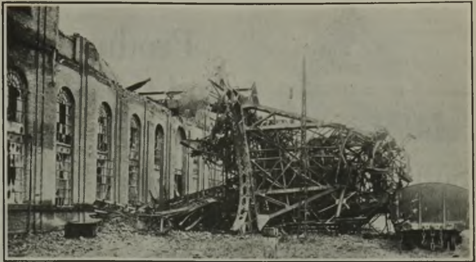
A Little of the Destruction Wrought by Germans at Notre Dame Colliery
