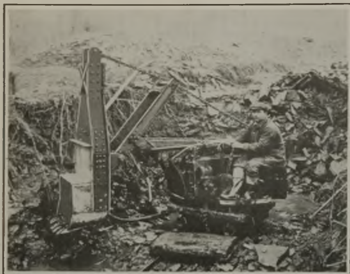
Mechanical Shovel Loading Rock from Open Cut
