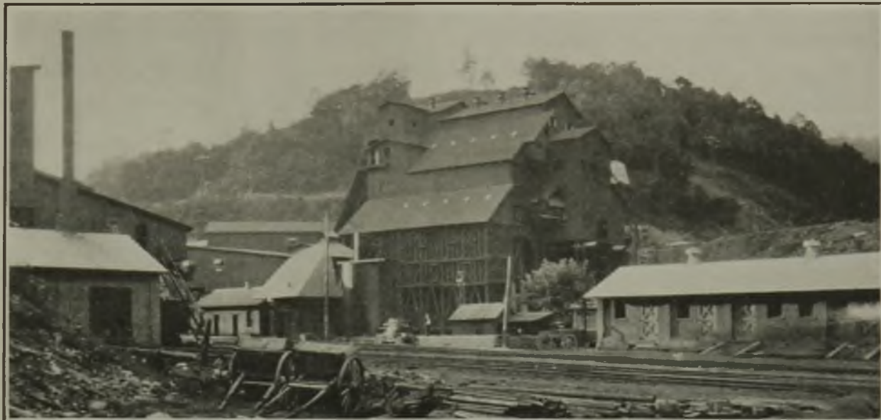
Crane Creek Tipple at McComas, W. Va.
