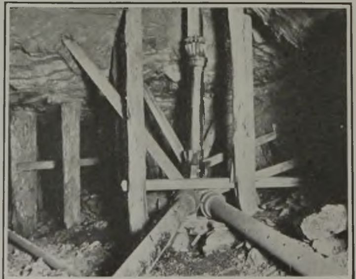
Flushing Pipe Entering Through Borehole
