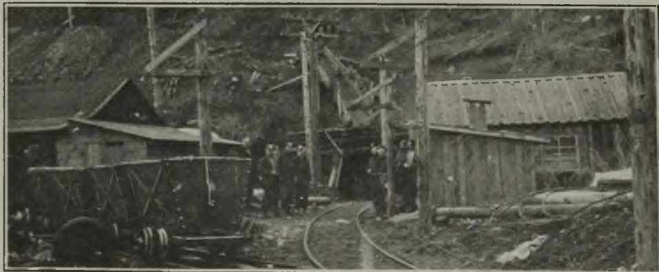
Entrance to Wilson Tunnel, Coalmont Collieries
