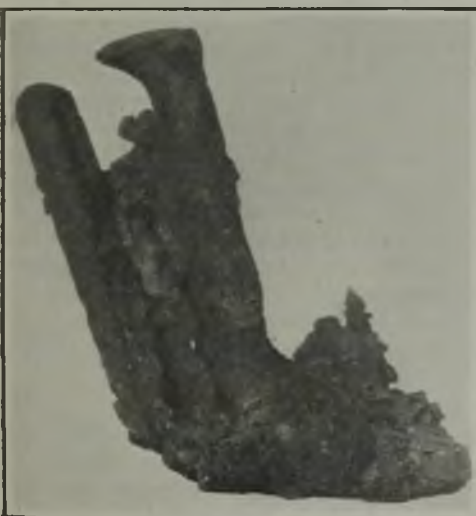
What Resulted from a Hasty Repair To a Resistance Bank
