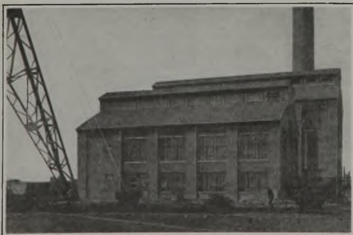
Power Plant at No. 4 Mine. Superior Coal Co.
