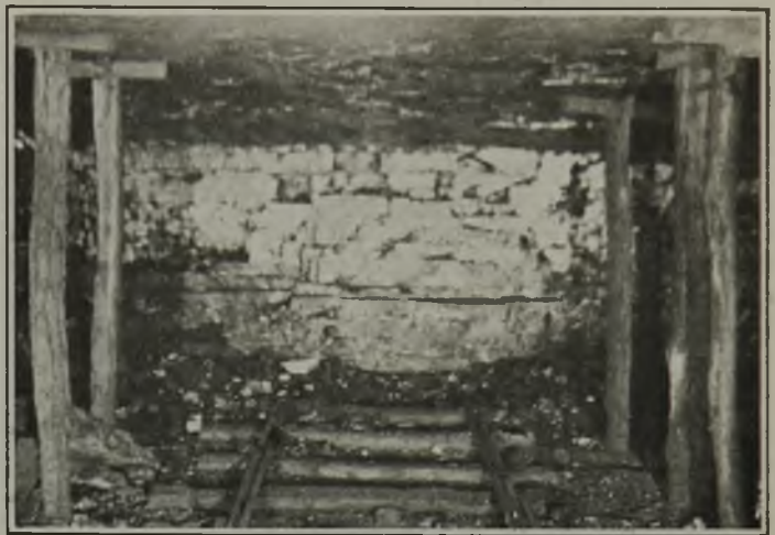
Fig. 2—Timbering Roof in Beech Bottom Mine
