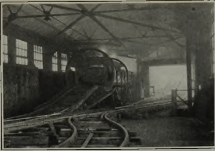
Fig. 5—Cars in Revolving Cradle Ready to Dump
