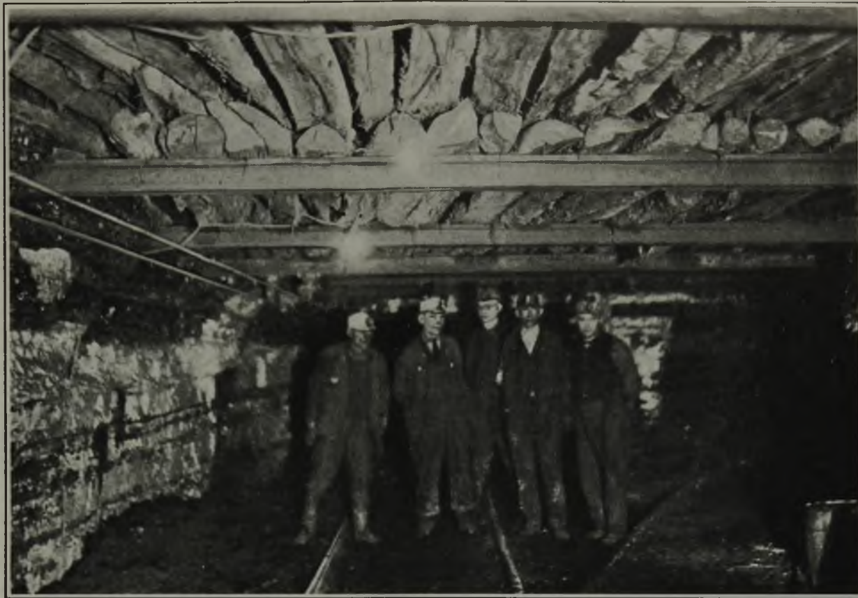
Careful timbering in Beech Bottom Mine, Power, W. Va.
