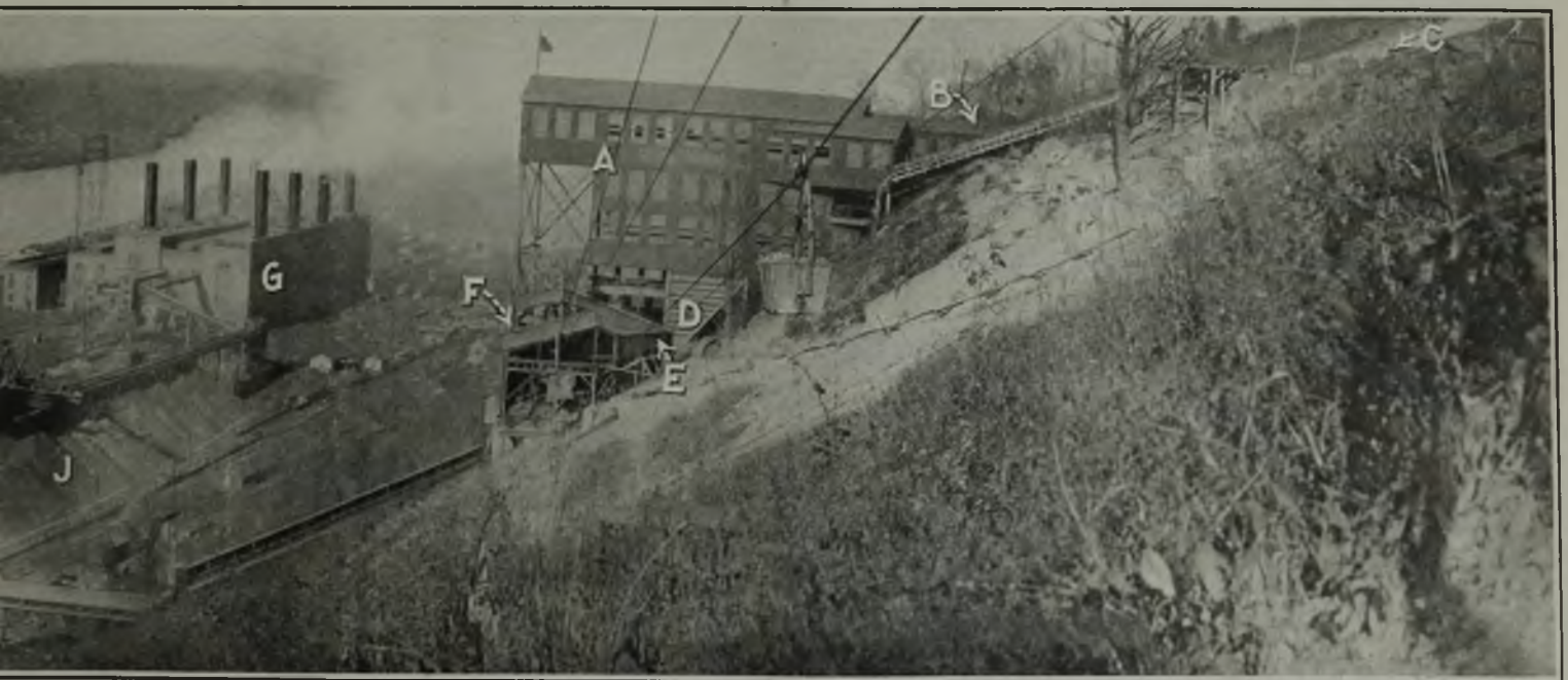
Bottom Mine Is Carried to the Power House and How the Rock Is Handled by an Aerial Tram E , aerial tramway for disposal of rock; F , crushers; G , power plant; H , machine shop and storehouse; J , river and rail delivery; N , discharge from railroad cars; M , delivery from river boats.
