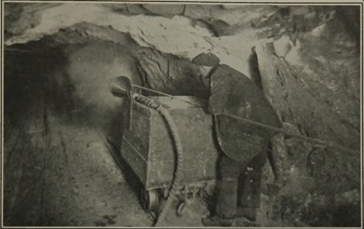
Stone Dusting by Compressed Air
