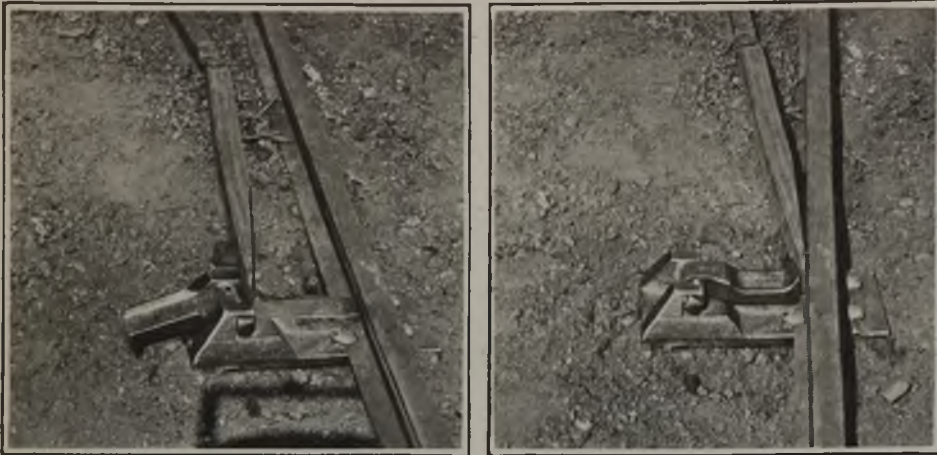
Fig. 13—A Switch Lock Installed
