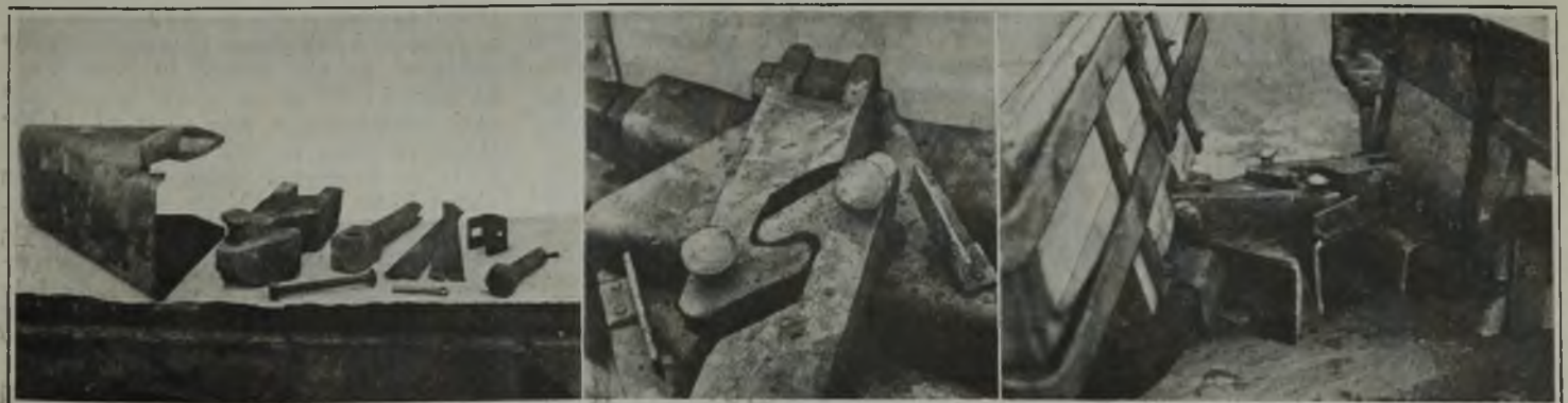
Fig. 16—Automatic Car Coupling and Its Parts
