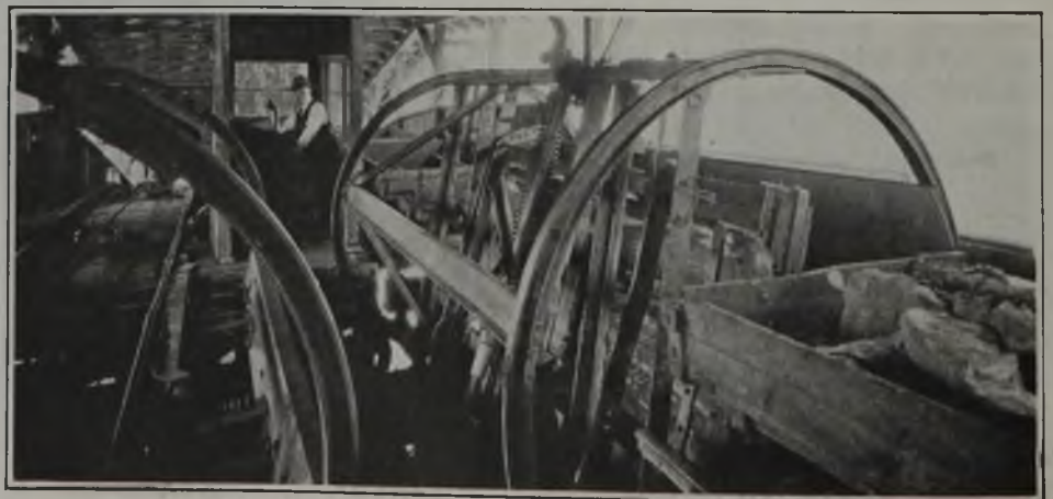
Fig. 14—Gravity Operated Rotary Dump
