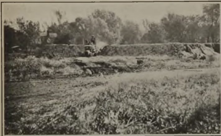
Fig. 2—Portable Elevator Loading Fired Coal
