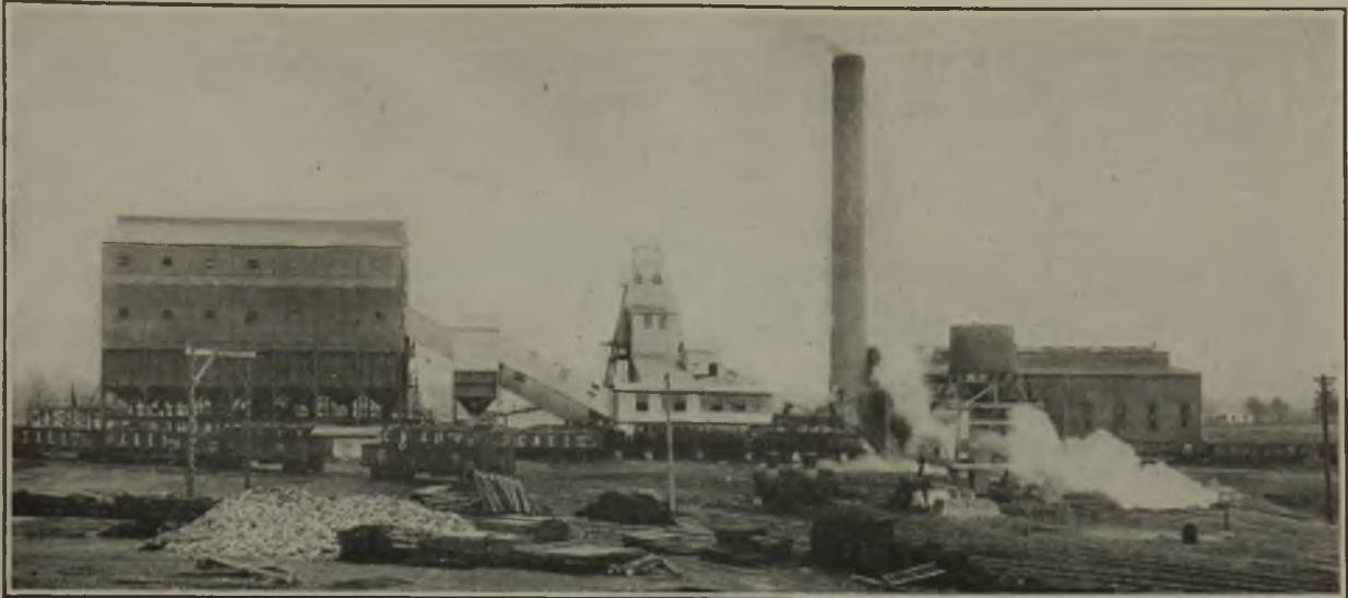
Surface Works of Old Ben No. 9 Mine
