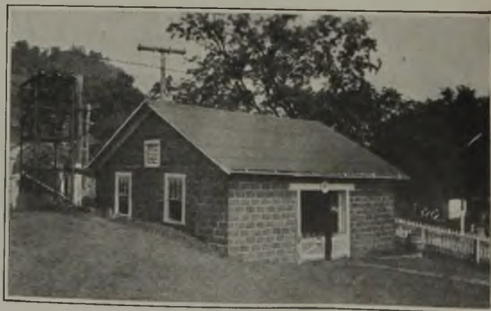
Fig. 6—A Well-Maintained Substation
