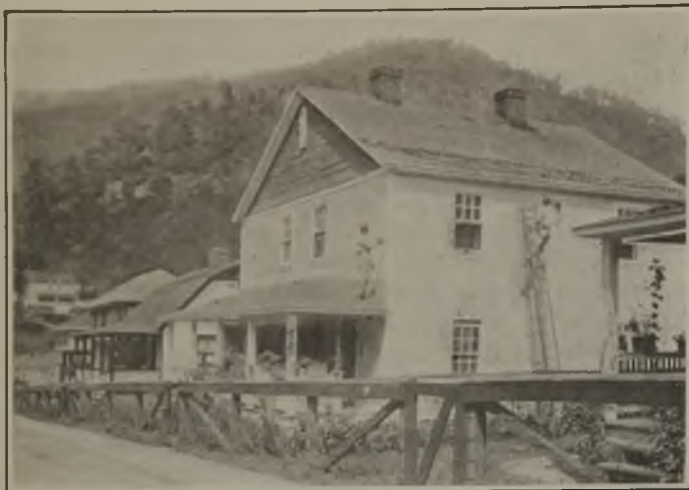
Fig. 5—Brushing on the Second Coat
