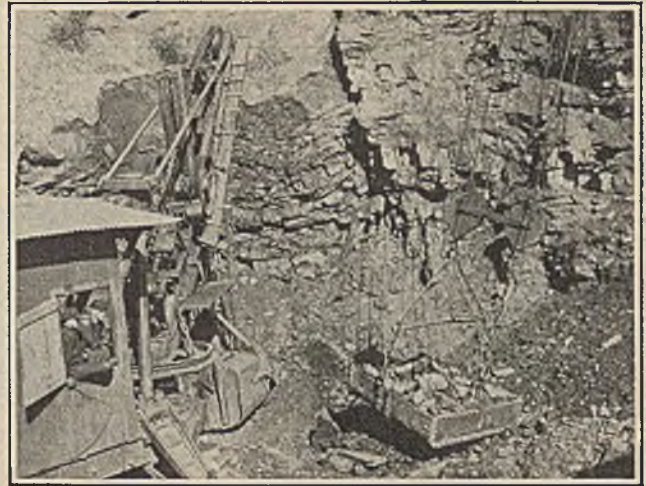
Fig. 3—Hoisting a Skip Load of Coal
