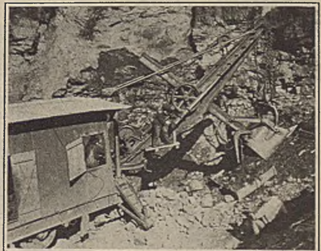
Fig. 1—Shovel Discharging to Cableway Skip
