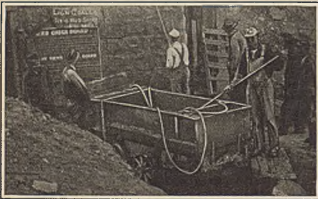
W. T. Reid Demonstrating Wet Adobe Spray
