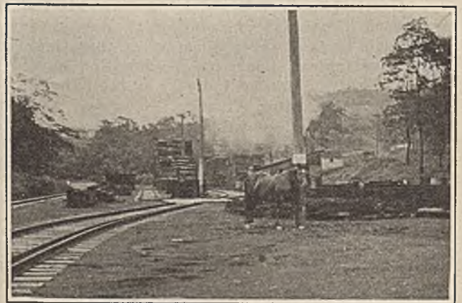
Supply Yard at Springdale Kept Neat and Clean
