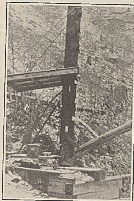
Locomotive Crab on Swing Derrick
