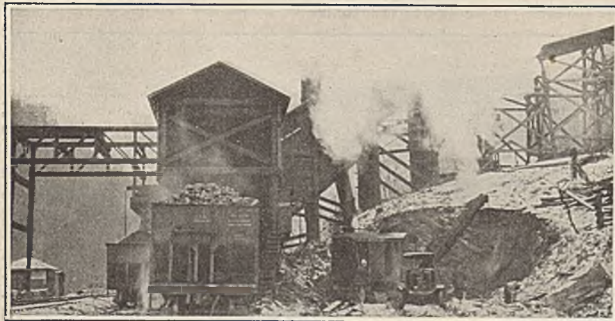
Clearing the Way for Two Additional Loading Tracks
