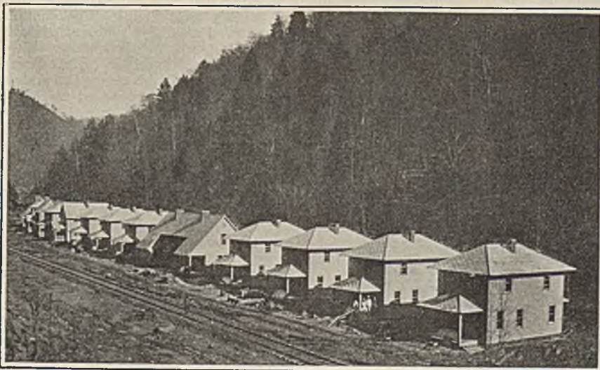
Houses Still Under Construction at Caretta, W. Va.
