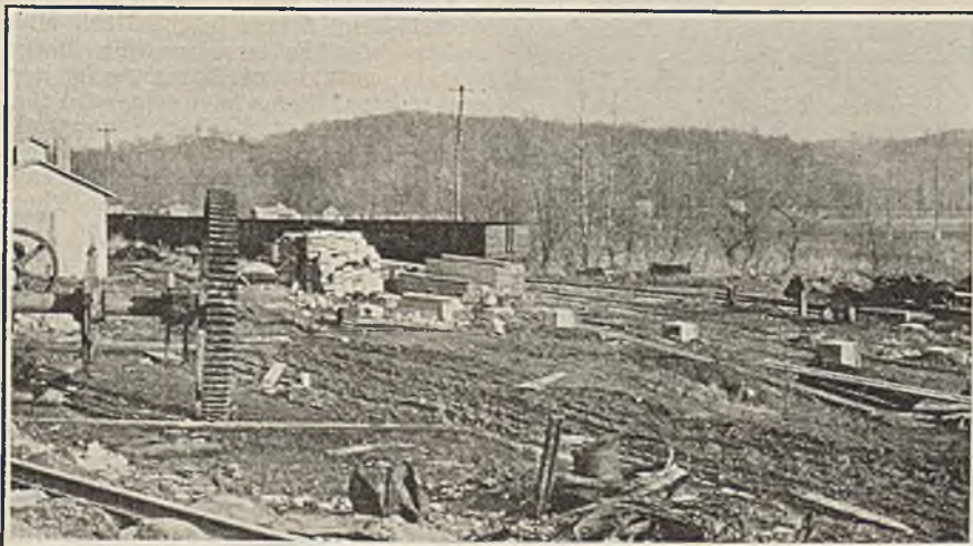
About to Replace Plant Destroyed by Fire
