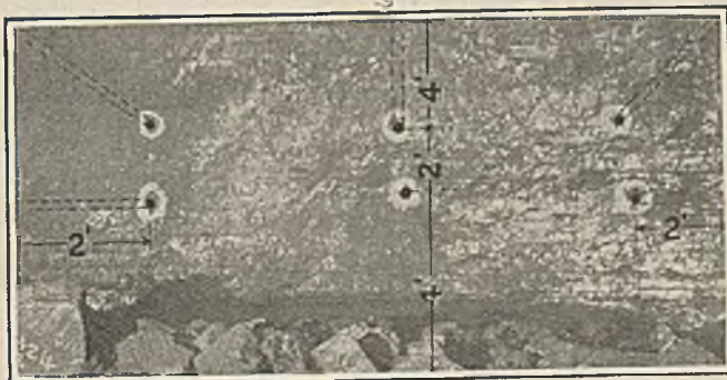
Fig. 9—Snub Cut Ready for Shooting
