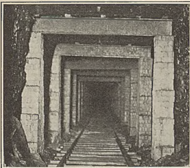
Fig. 1—Brick Pillars and Heavy Beams, Corning, Ohio
