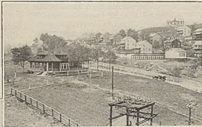
Right—Home of Division Superintendent with a Part of Barrackville Village in the Rear Background.
