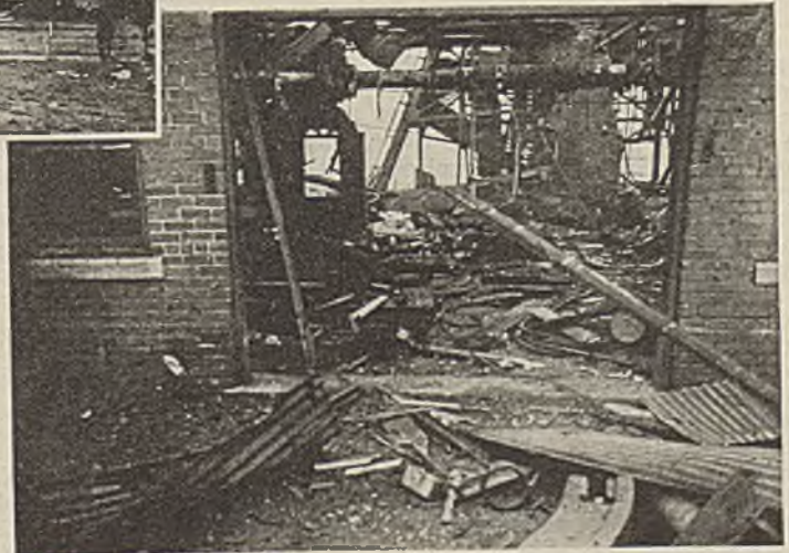
Right — Compressor Room. The Explosion Was So Violent That This Outside Structure, Which Was Being Converted Into a Bathhouse, Was Almost Entirely Demolished.
