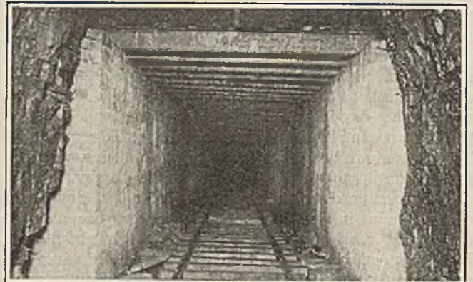
Fig. 2—Bridge Under Railroad and River, Corning, Ohio
