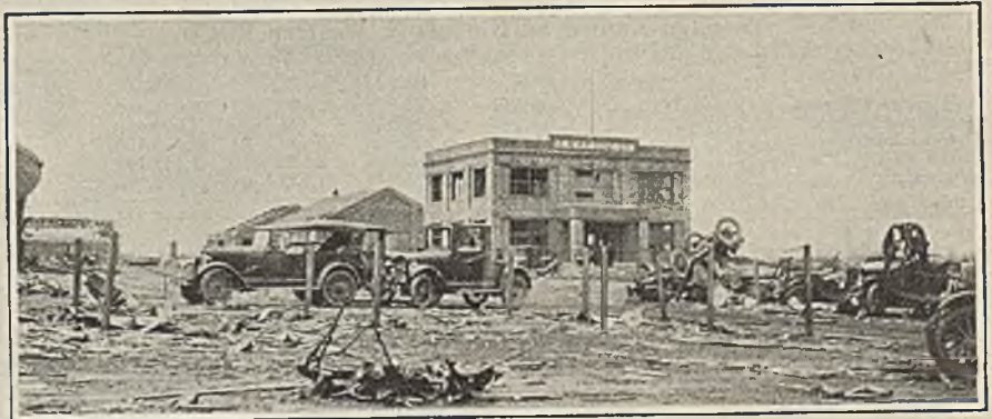
New Orient Office Building Stood Firm
