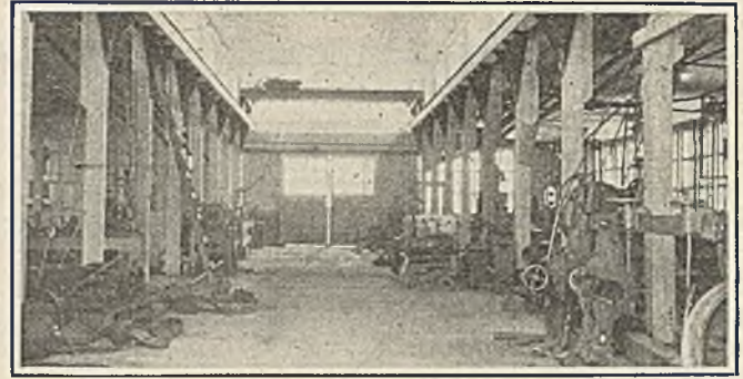
Fig. 2—Central Bay of Shop Interior
