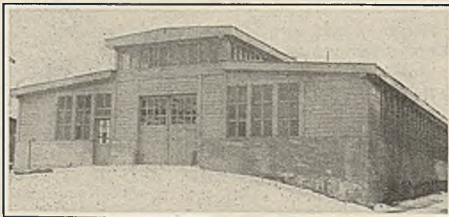
Fig. 1—Exterior of New Shop Building
