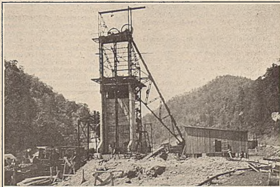
Man Shaft at Consolidation Coal Co.'s Mine Caretta, W. Va.
