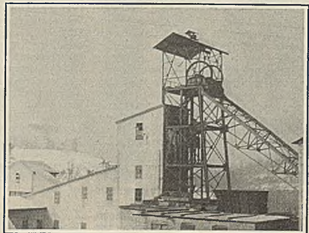
Steel Headframe and Tipple, Cranberry No. 1 Mine
