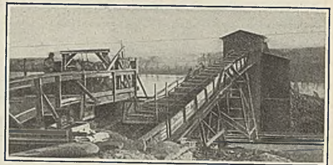
Fig. 2—Car Dump and Conveyor to Breaker
