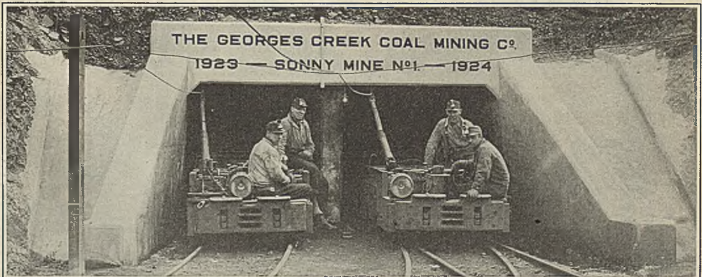
Main Entry Portal of Sonny Mine Where Louis F. Gerdetz Has Applied His Mining System Effectively Although the mine is operating in an old property which was abandoned years ago, the enormous tonnage of high quality coal remaining will take years for complete recovery. Consequently that part of the main heading under extremely light cover is supported by reinforced concrete. These locomotives are 8-tonners and combine trolley, crab-reel and cable-reel types. They serve on the main hauls as well as in gathering loads from the faces:
